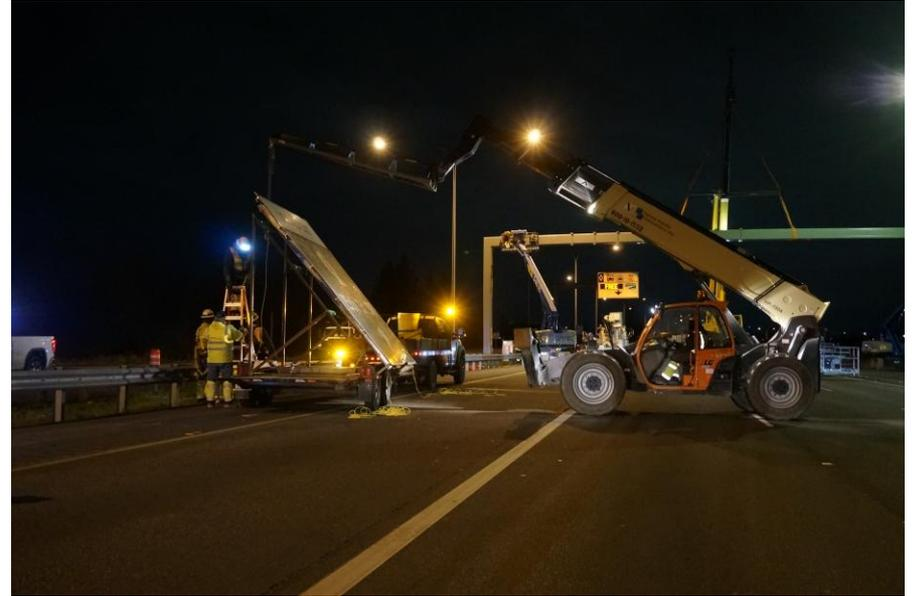
*Crews hoisting a new guide sign on to a new sign structure.*
