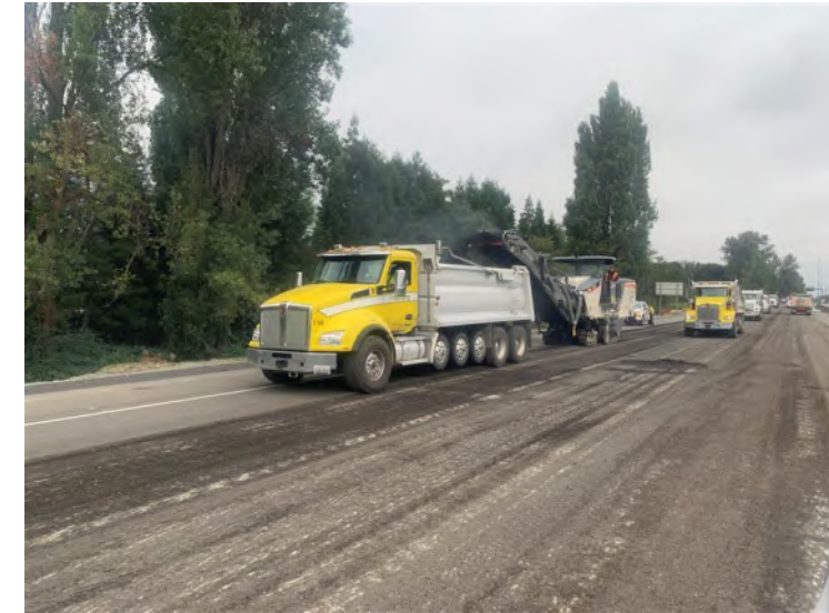
Repaving on SR 167
