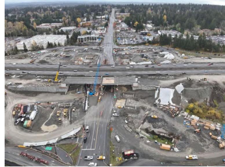
NE 85 th St interchange construction
