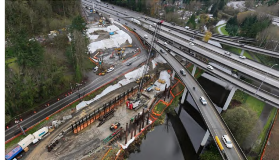
I-405/SR 522 interchange construction
