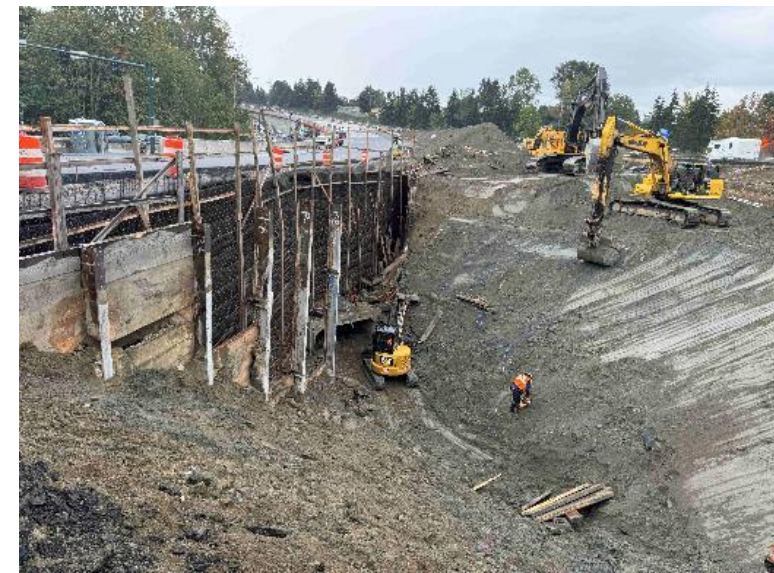
Culvert replacement near Coal Creek
