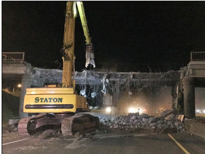
Removing concrete structures over SR 520
