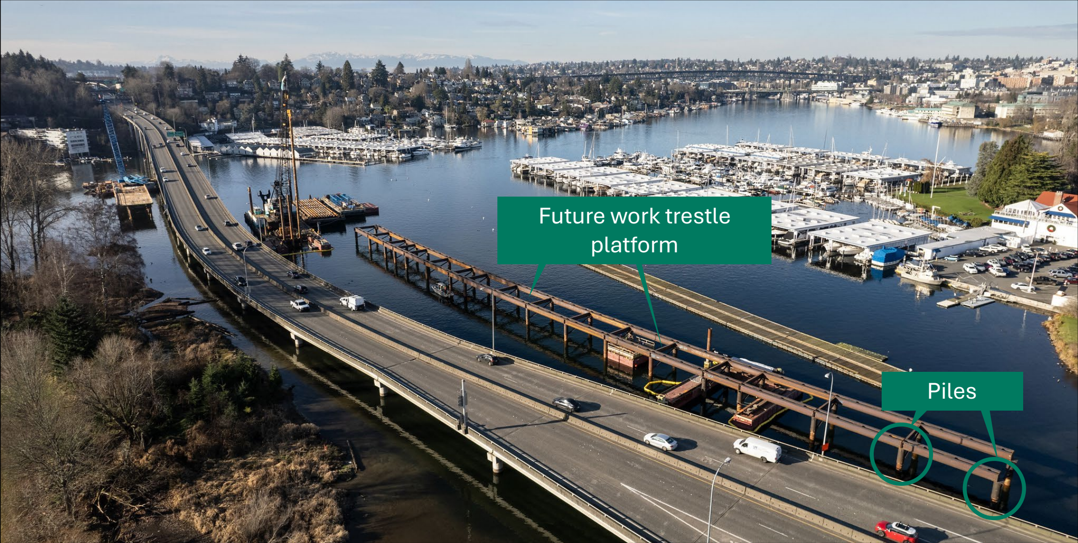
Crews have installed piles in Portage Bay to support the temporary work trestle.
