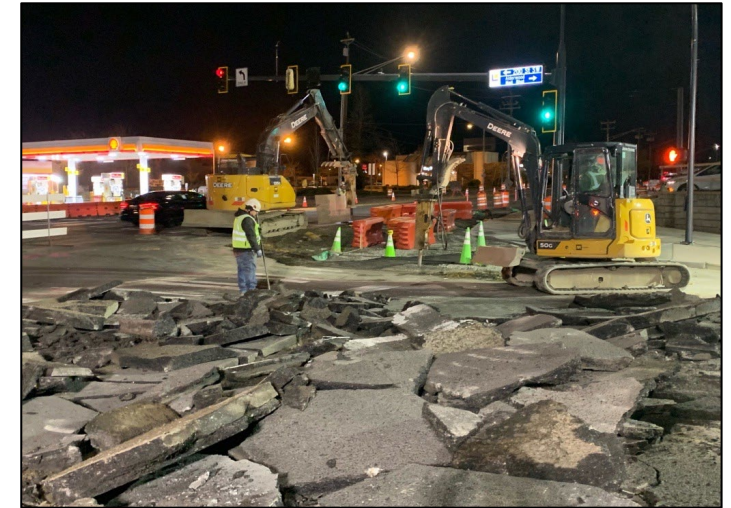
Removing concrete roadways
