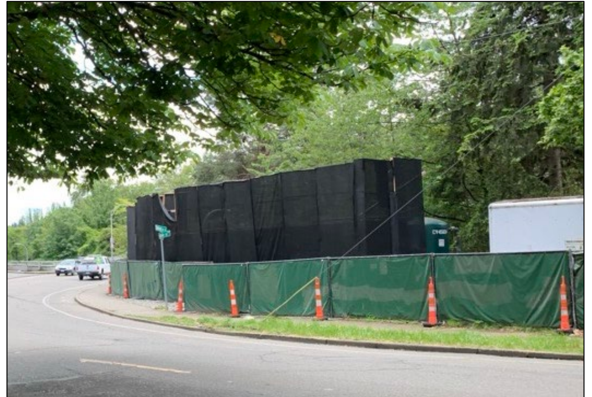
Photo of an Acoustifence®, a common type of acoustic fence.
