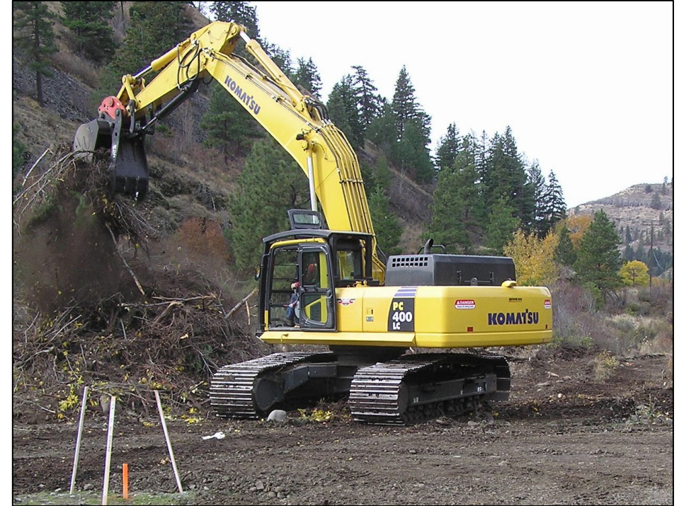
An example of machinery used to remove trees.
