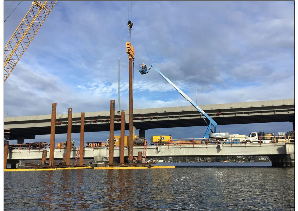
A vibratory hammer used during construction of the SR 520 Floating Bridge.
