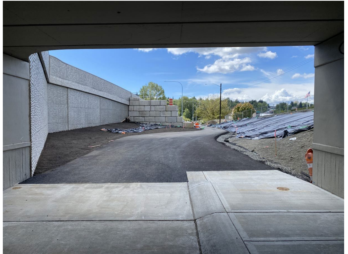
West entrance to the tunnel under Montlake Boulevard (May 23)
