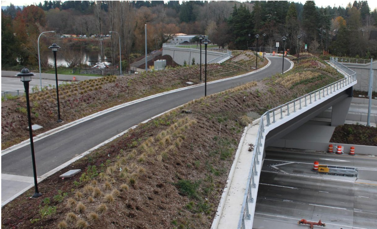
Bicycle and pedestrian bridge deck (Dec 5)
