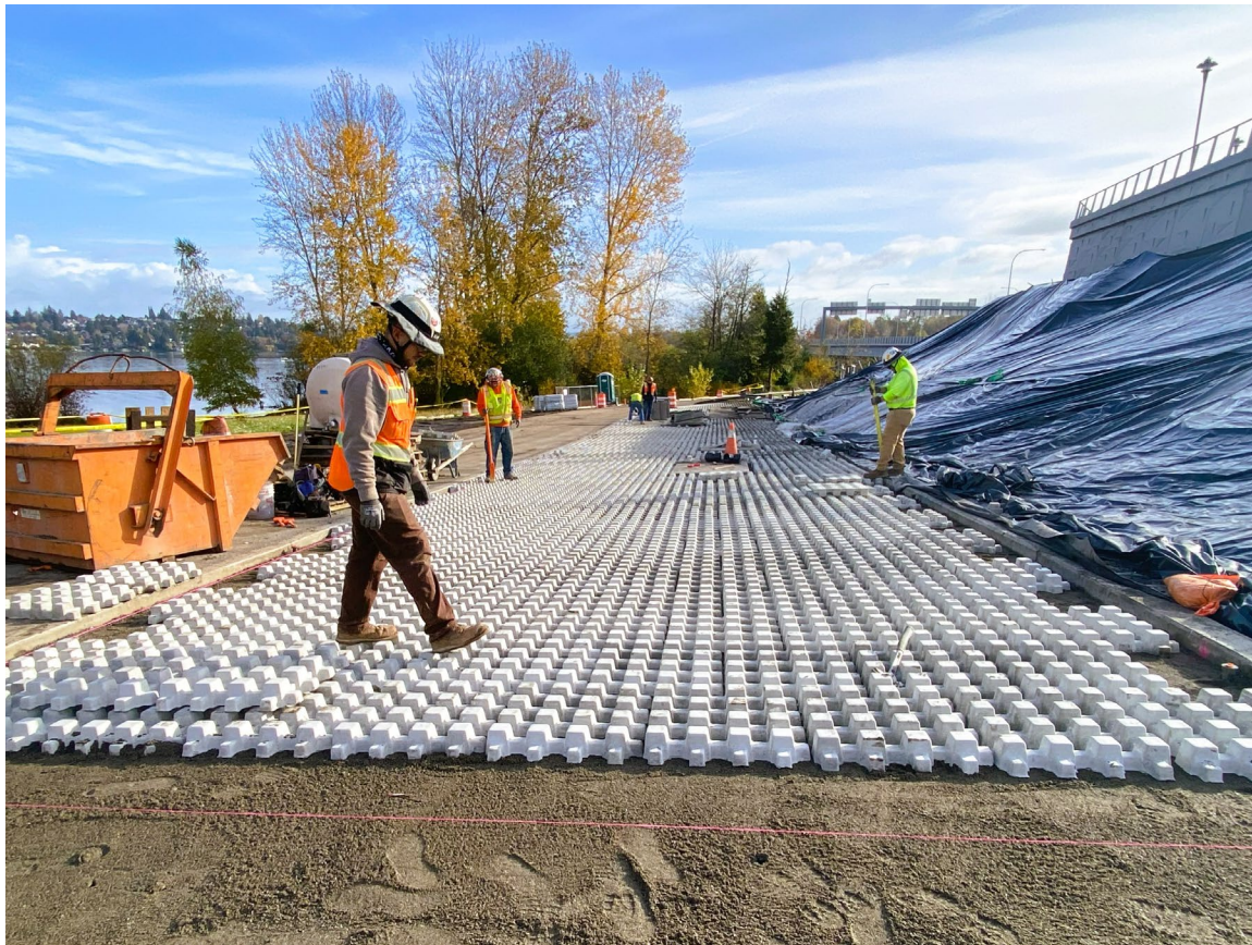
Grass paver installation (November 1)
