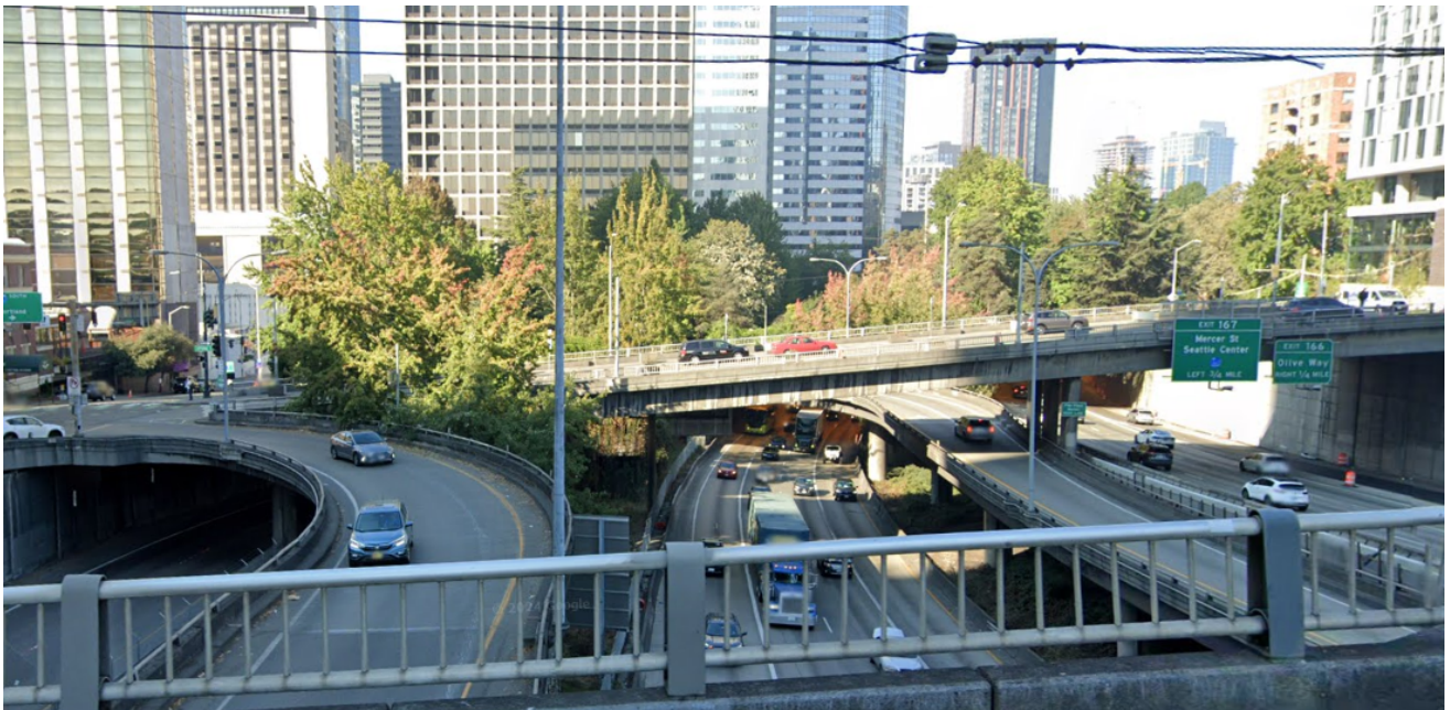
Figure 9. Complex Network of I-5 Ramps, Travel Lanes, Collector-Distributor Roads, and Overcrossings
