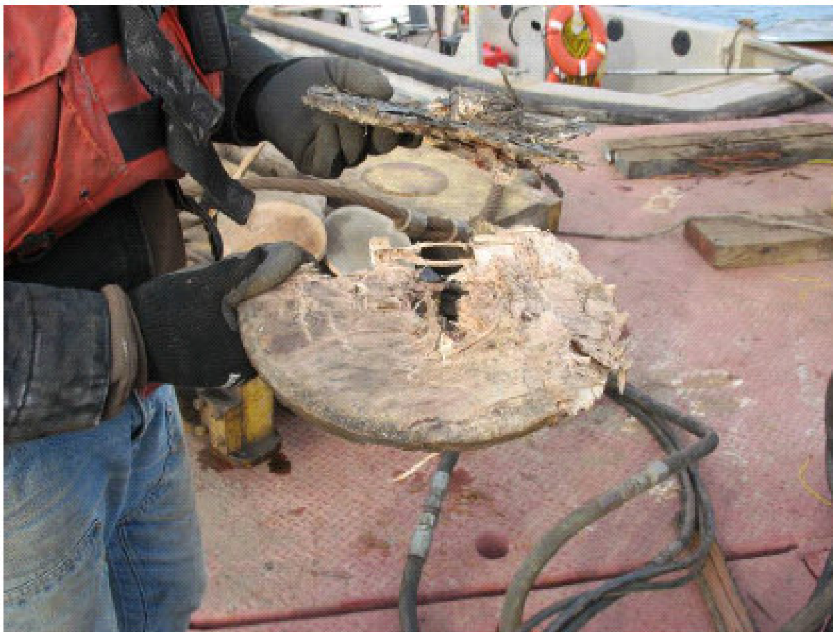
Figure 7: Fractured and compressed wood pile cap after being used on piles 5, 6, and 7 (photo courtesy of Washington State Parks and Recreation, R. Johnson)
