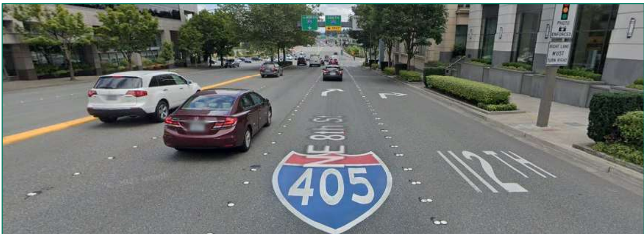
Painted directional shields on pavement: Navigational symbols or markings painted directly onto road surfaces. They serve as supplemental information for overhead and side-mounted signs, offering additional guidance to drivers. Pictured above: Painted directional shields on pavement on NE 8 th Street in Bellevue.
