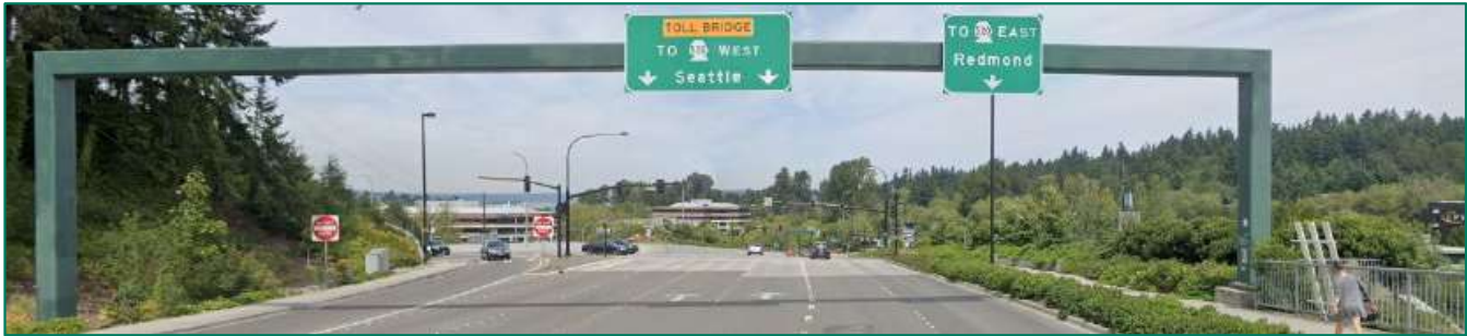
Sign bridge: Structure supporting signs spanning across a roadway. Pictured above: Sign bridge over Lake Washington Boulevard in Bellevue.
